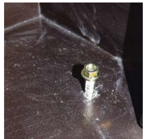
The dynabolts will need to be tapped into the hole with a hammer, but it is important to do this with the nut lightly screwed on to prevent losing the bolt down the hole.
